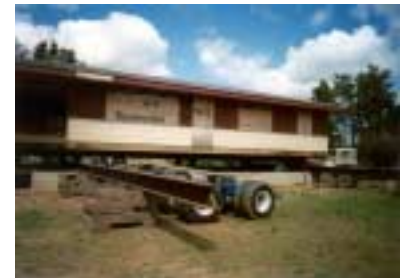
Figure 1-1: Relocating flood prone structure
